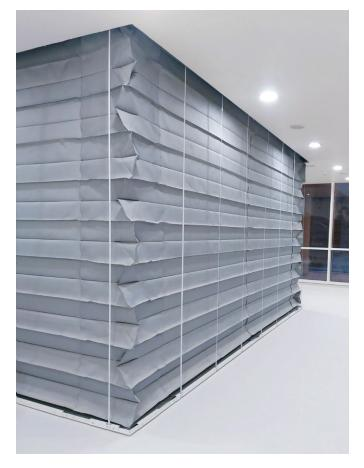
NAFFCO Melodeon Fire Curtain systems prevents the spreading of fire from one area to another. The Curtain assembly comprises fire-rated fiberglass fabric uniquely folded into a compact head box that is typically installed above the ceiling with a finished bottom tray. This makes the system virtually invisible until activated. The curtain descents at a controlled speed upon receipt of signal from a fire alarm and provides fire integrity for up to four hours\*.
