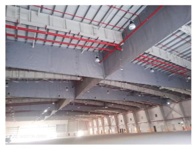
NAFFCO Static Smoke Curtains are a reliable solution for offering smoke protection in commercial and industrial buildings. Draft curtains, which are secured to structural steel, ensure that smoke and hot gases emitted during fire remain buoyant within the smoke zone, in accordance with smoke management strategies.
