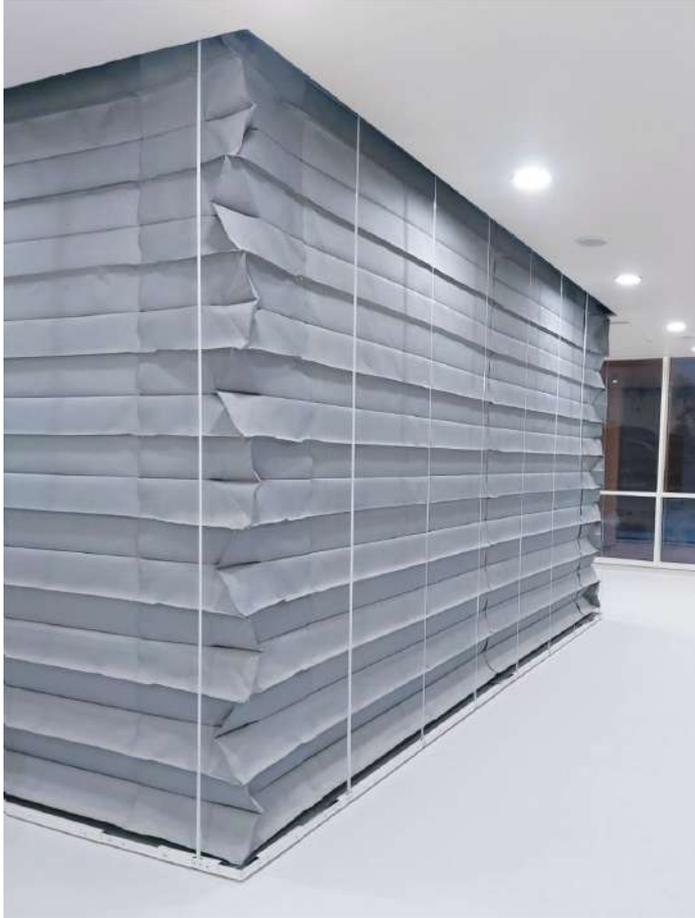
NAFFCO Accordion Fire Curtain systems prevent the spreading of fire from one area to another. The Curtain assembly comprises fire-rated fiberglass fabric uniquely folded into a compact head box that is typically installed above the ceiling with a finished bottom tray. This makes the system virtually invisible until activated. The curtain descends at a controlled speed upon receipt of signal from a fire alarm and provides fire integrity for up to four hours\*.
