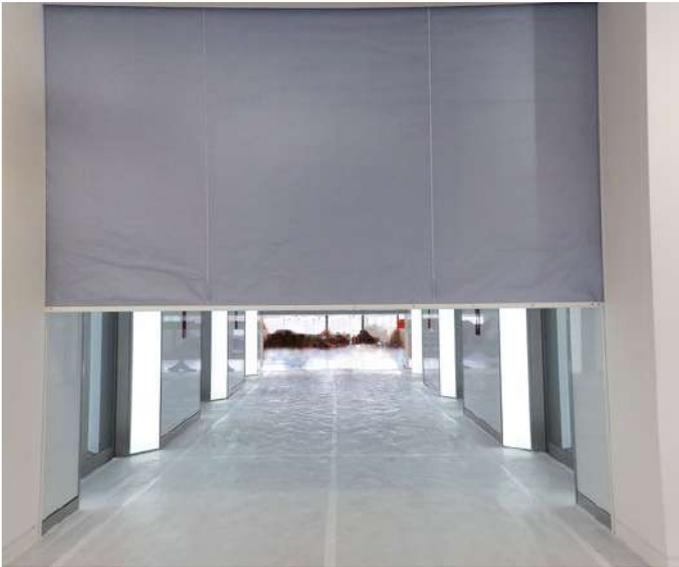
Fire containment systems prevent the spreading of smoke from one zone to another. NAFFCO curtain comprises of flexible heat resistant fabric with fire integrity up to 240mins\*. The tube contains a DC electric motor which holds the curtain retracted at ceiling level at all times and deploys upon the receipt of fire alarm signal. The bottom bar ensures safe and controlled descent of the curtain with gravity fail safe.
